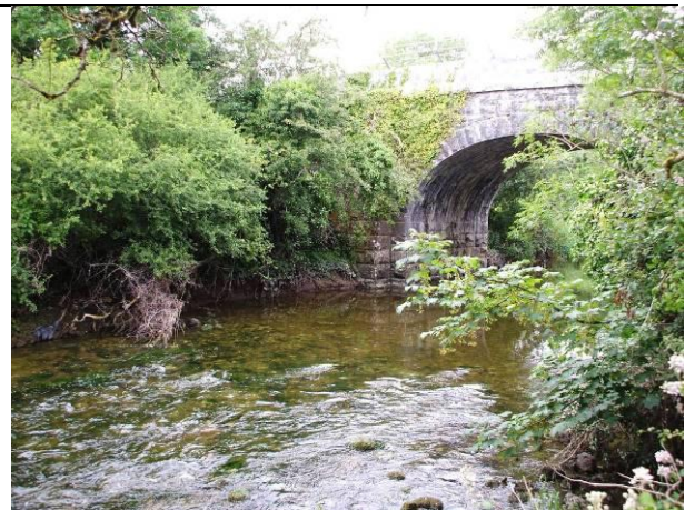
Plate 44: View US over shallow riffle /run downstream from the masonry railway bridge (Point 48) (20-7-2011).
