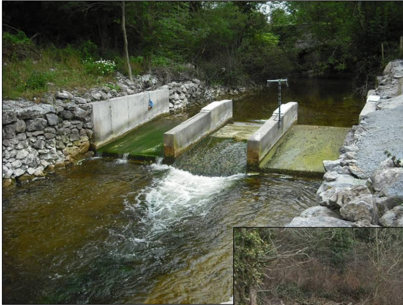
Photographs No. 22 and 23 Existing Salmon Counter
