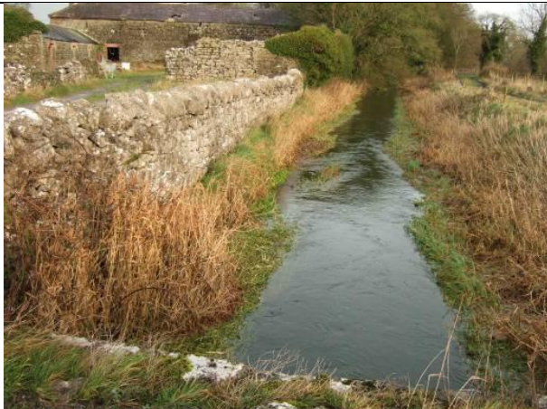
Plate 69: View d/s from farm road bridge at AG11 (8-1-2012)
