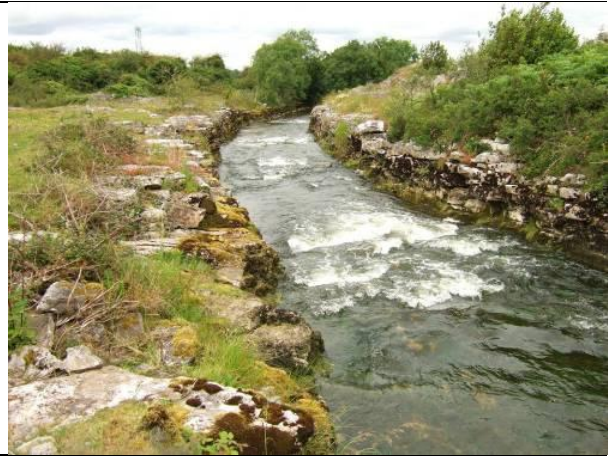
Plate 26: Much more closely spaced step/weir/run sequences near Point 27 between Dunkellin Bridge and Rinn Bridge. (21-7-2011)
