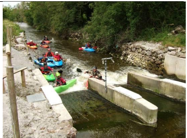
Plate 8: Salmon counter below Killeely Bridge - view downstream. (20-7-2011)
