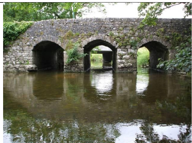
Plate 48: View upstream over shallow glide/run towards old bridge at Craughwell, with the N6 Bridge visible beyond. Crayfish were abundant under boulder/cobble in this stretch.
