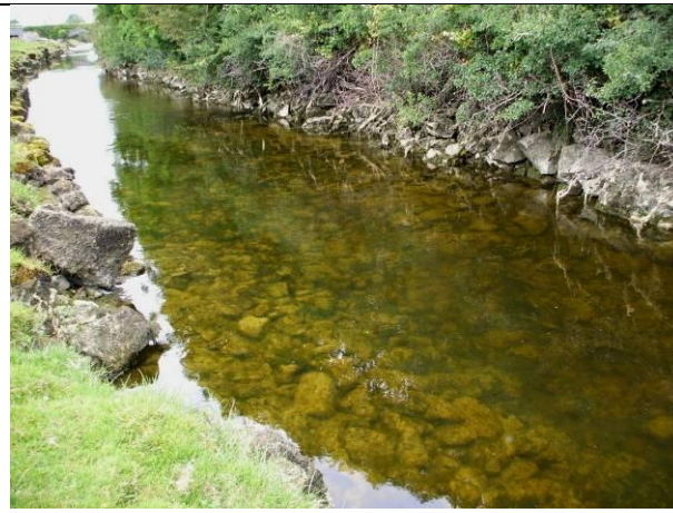
Plate 20: Shallow, narrow glide upstream of Dunkellin Bridge- note coarse substrate with rock cut banks on true right and rip-rap reinforcement on true left(21-7-2011)
