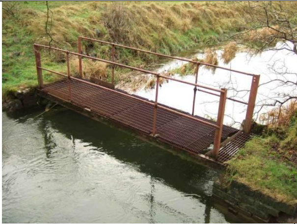
Plate 67: Metal footbridge at AG 10 - view u/s (8-1-2012)
