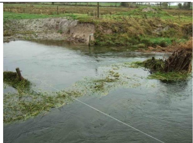
Plate 64: View u/s at AG8 - cattle access point (8-1-2012)
