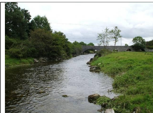
Plate 17: View upstream towards Dunkellin Bridge over shallow run / glide (20-7-2011).
